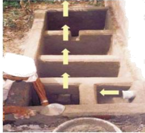
Construction of greywater treatment system
